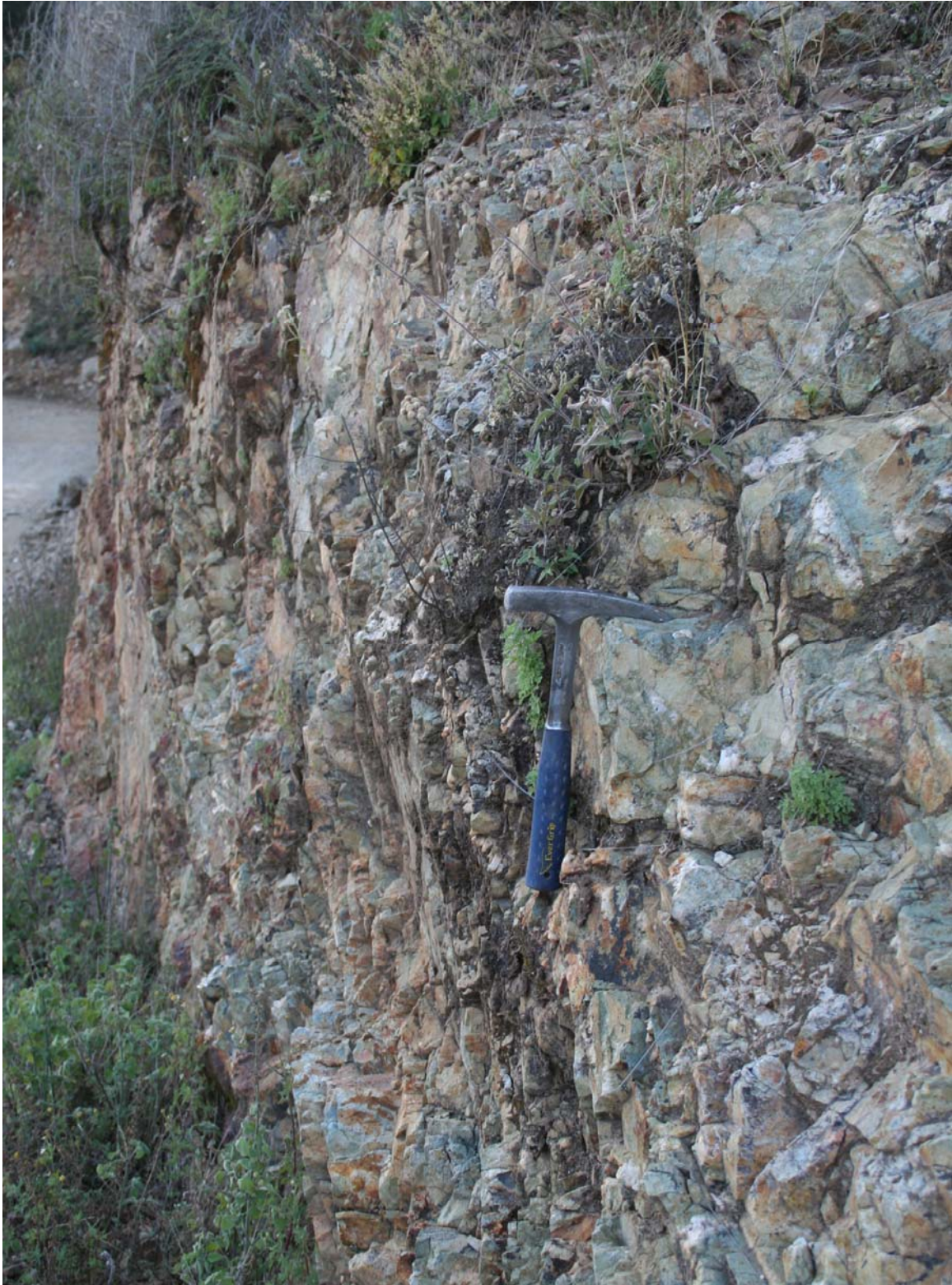
Figure 13. La Incredible crackle breccia, looking S70W along main fracture direction cutting andesite. Coarse crystalline quartz fills voids. Alteration is silica-epidote-chlorite, with strong limonite and Cuox staining.
